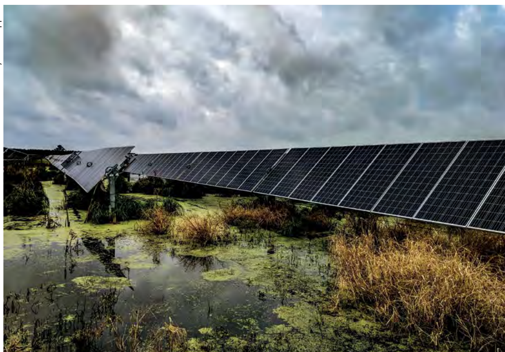
Courtesy Solar support
